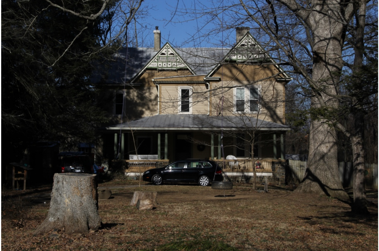
William Worley House (former C. G. Worley House), 1 Worley Place, façade, view to northwest
