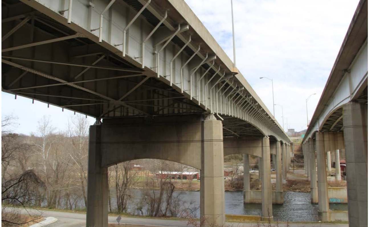
Great Smoky Mountain Park Bridge, view to northeast across Emma Road
