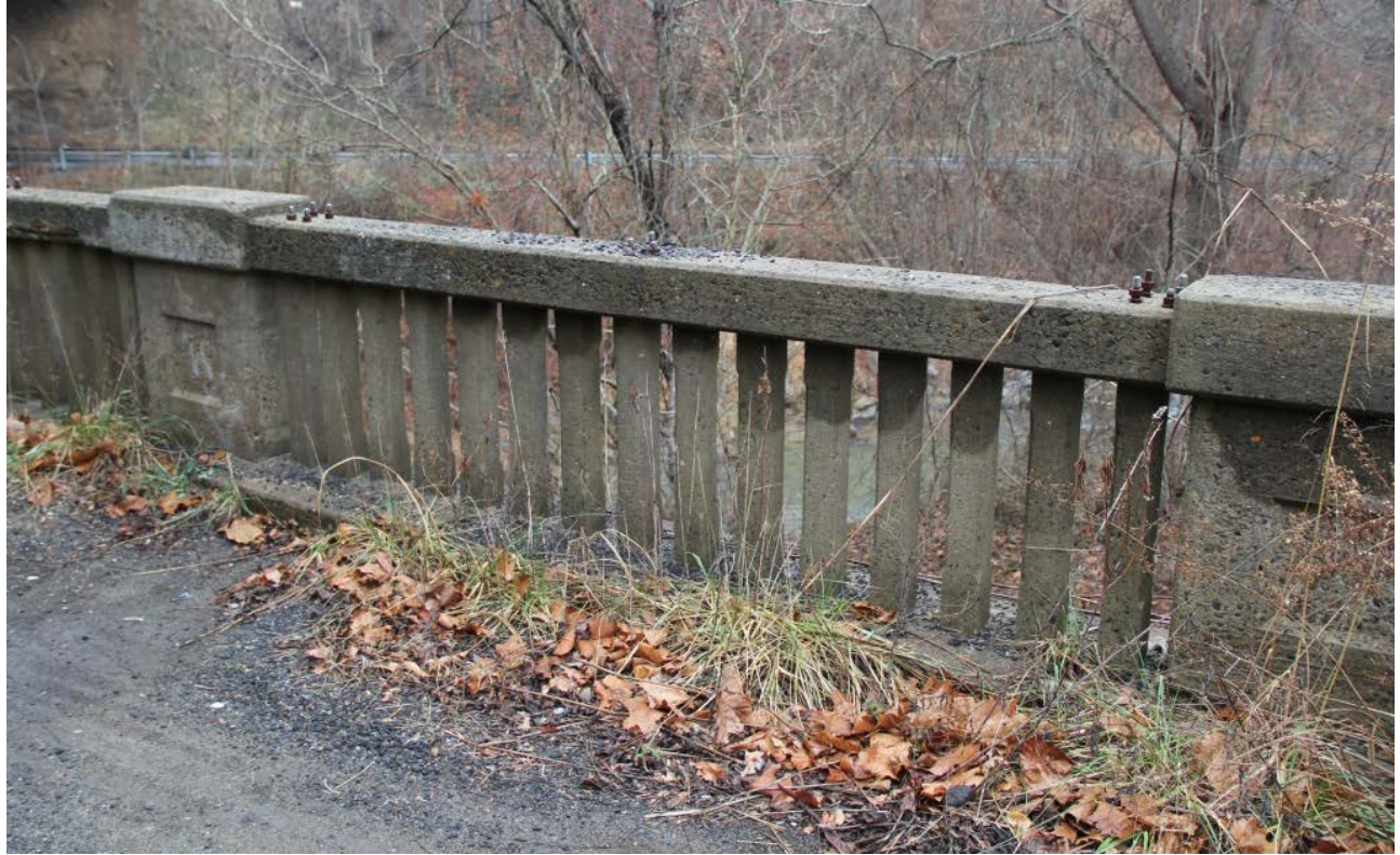
Bridge No. 216, southeast railing, balustrade detail, view to east
