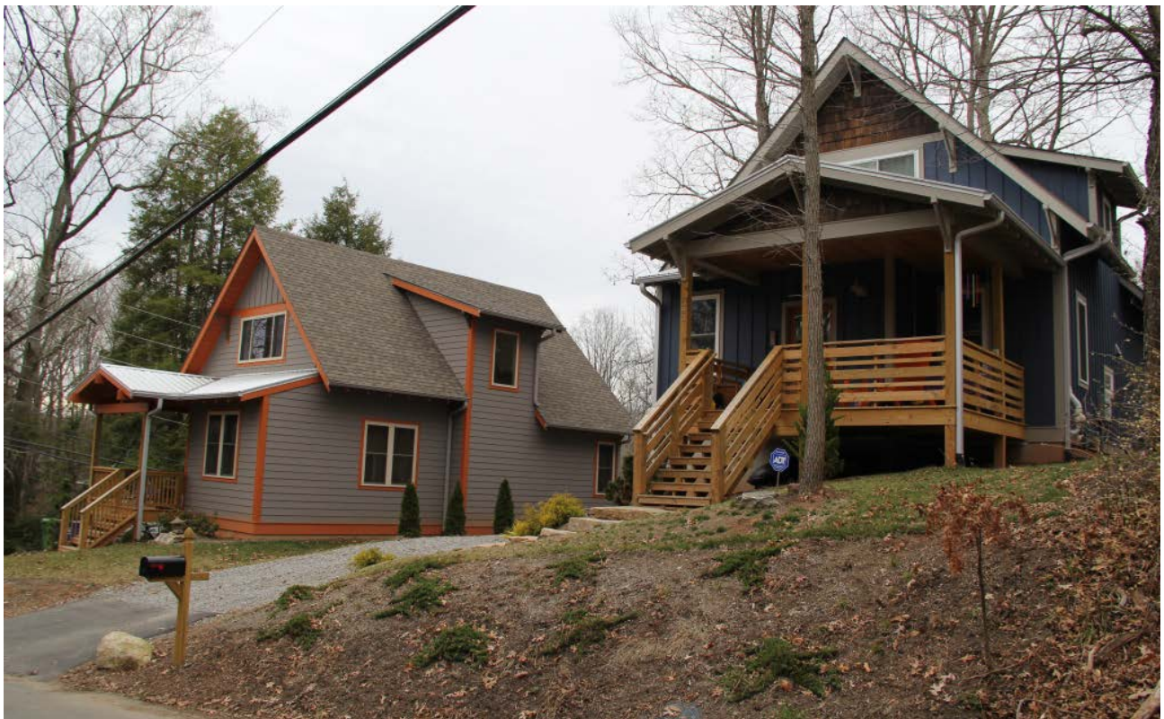
Houses, built 2013, 383 & 387 Pearson Drive, view to west (excluded from boundary expansion)
