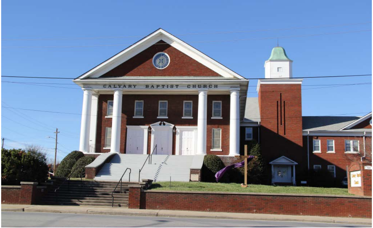
Calvary Baptist Church, façade, view to north
