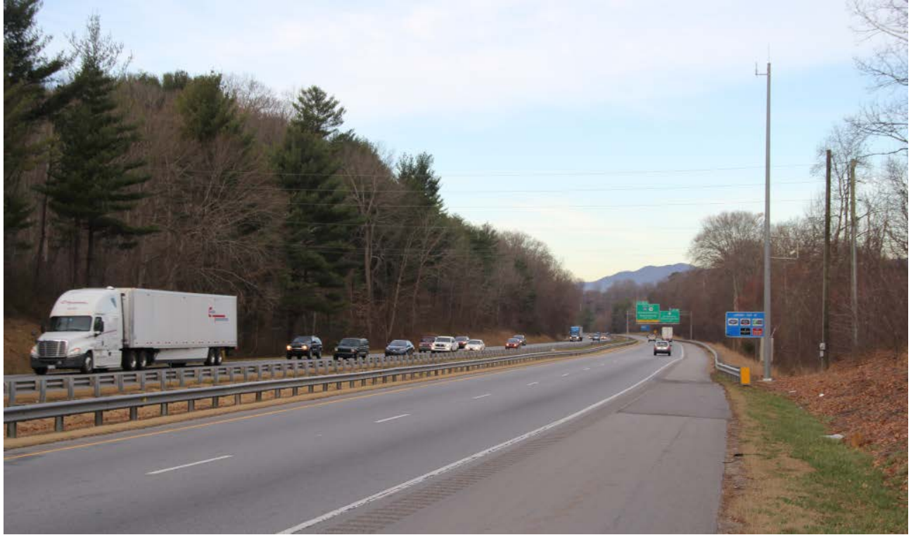
I-40 through Biltmore Estate, view to west at mile marker 48
