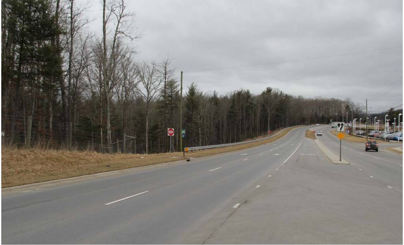
Brevard Road (NC 191) adjacent to Biltmore Estate, view to southwest
