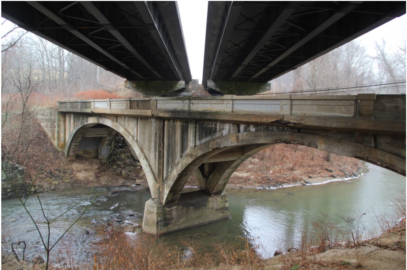
Bridge No. 216 over Hominy Creek, view to west
