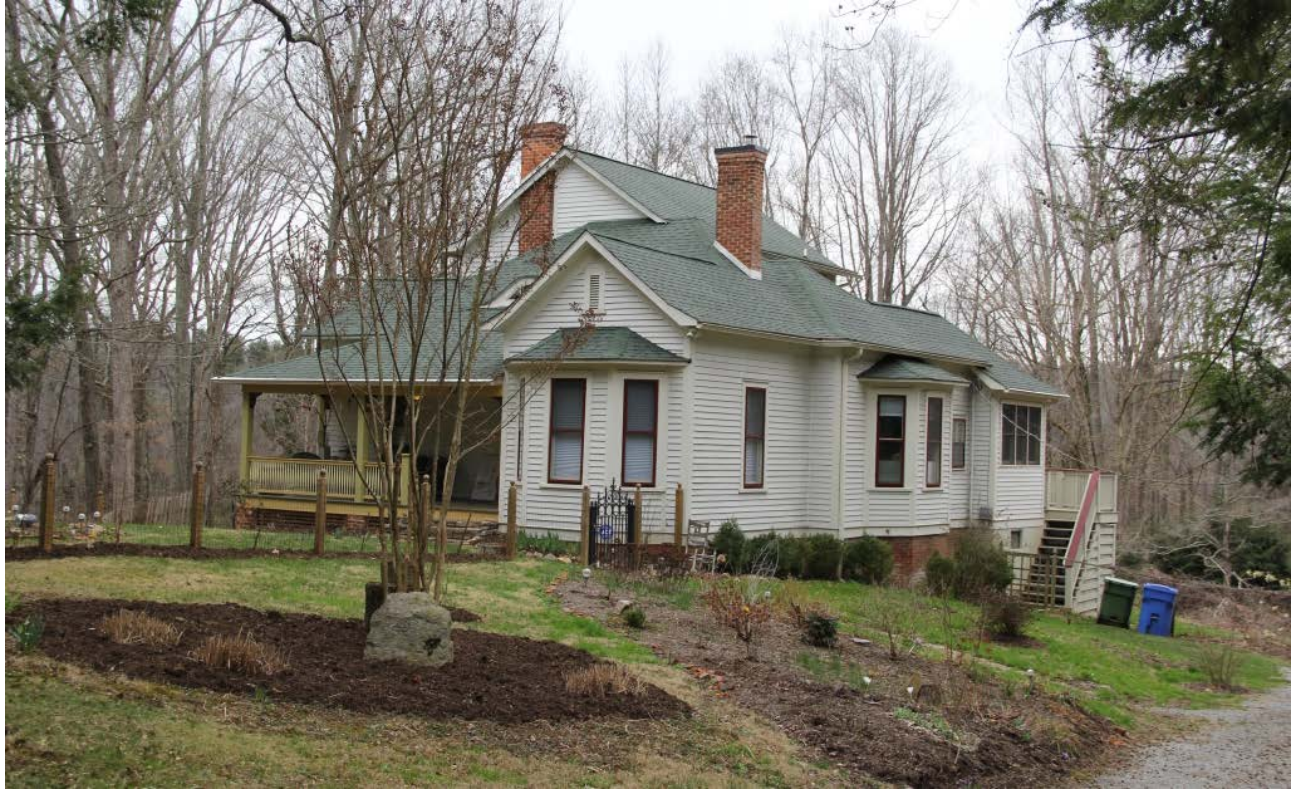
House, 403 Pearson Drive, view to northwest
