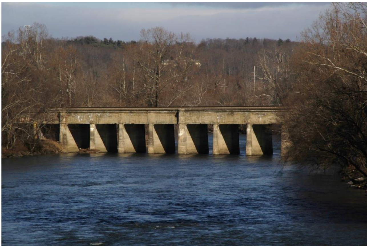
Southern Railroad Bridge over French Broad River, view to south
