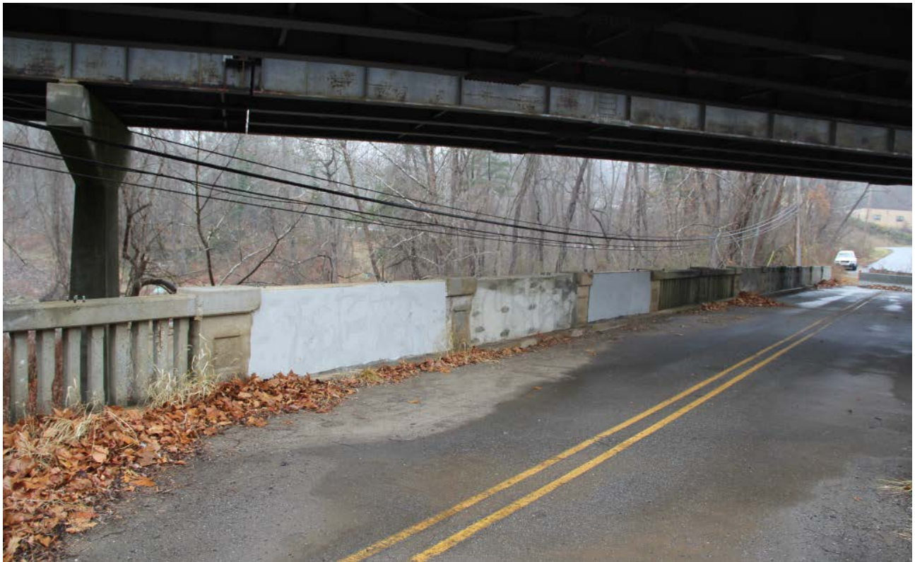
Bridge No. 216, northwest railing, view to north
