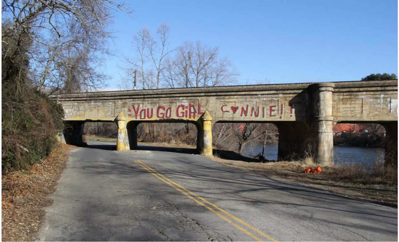
Southern Railroad Bridge over Emma Road, view to north
