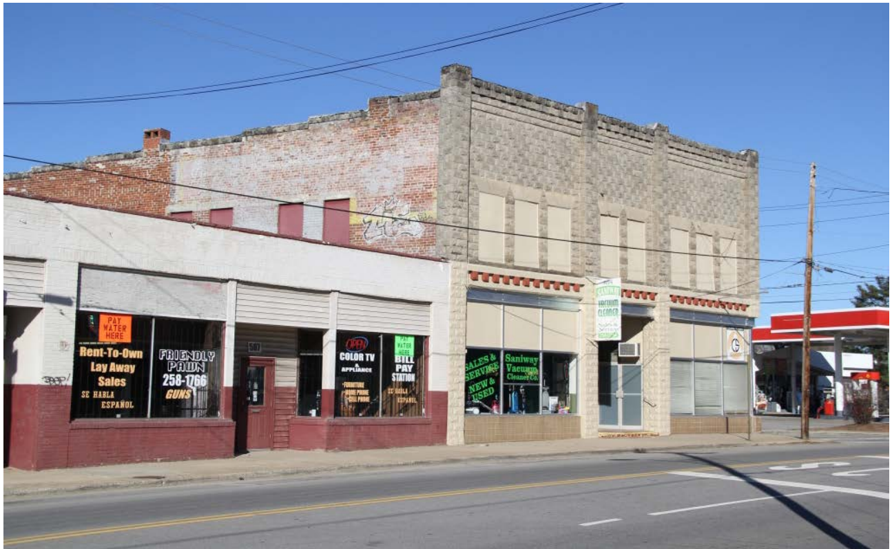
Baker Building, oblique front view to northeast
