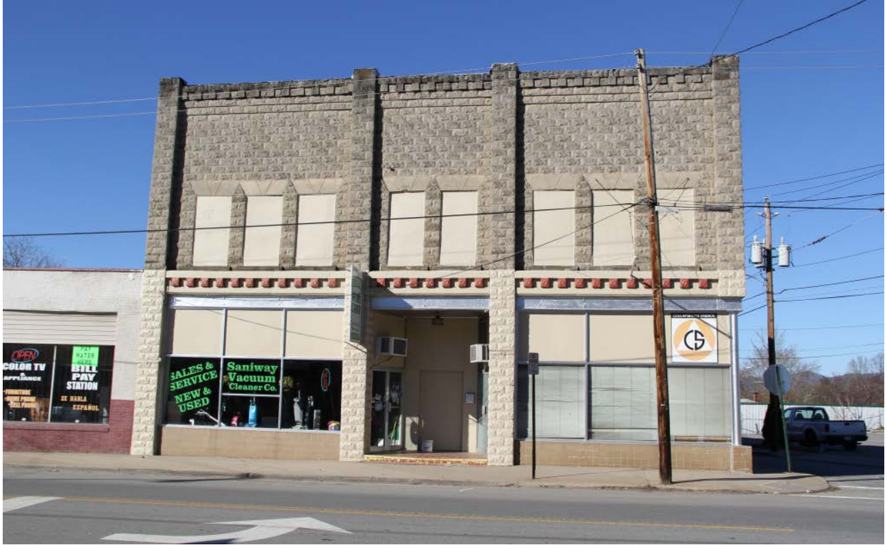
Baker Building, facade, view to north
