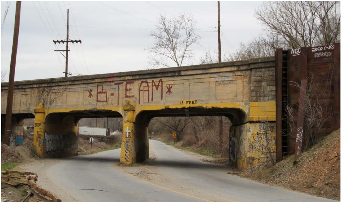
Southern Railroad Bridge over Riverside Drive, view to north
