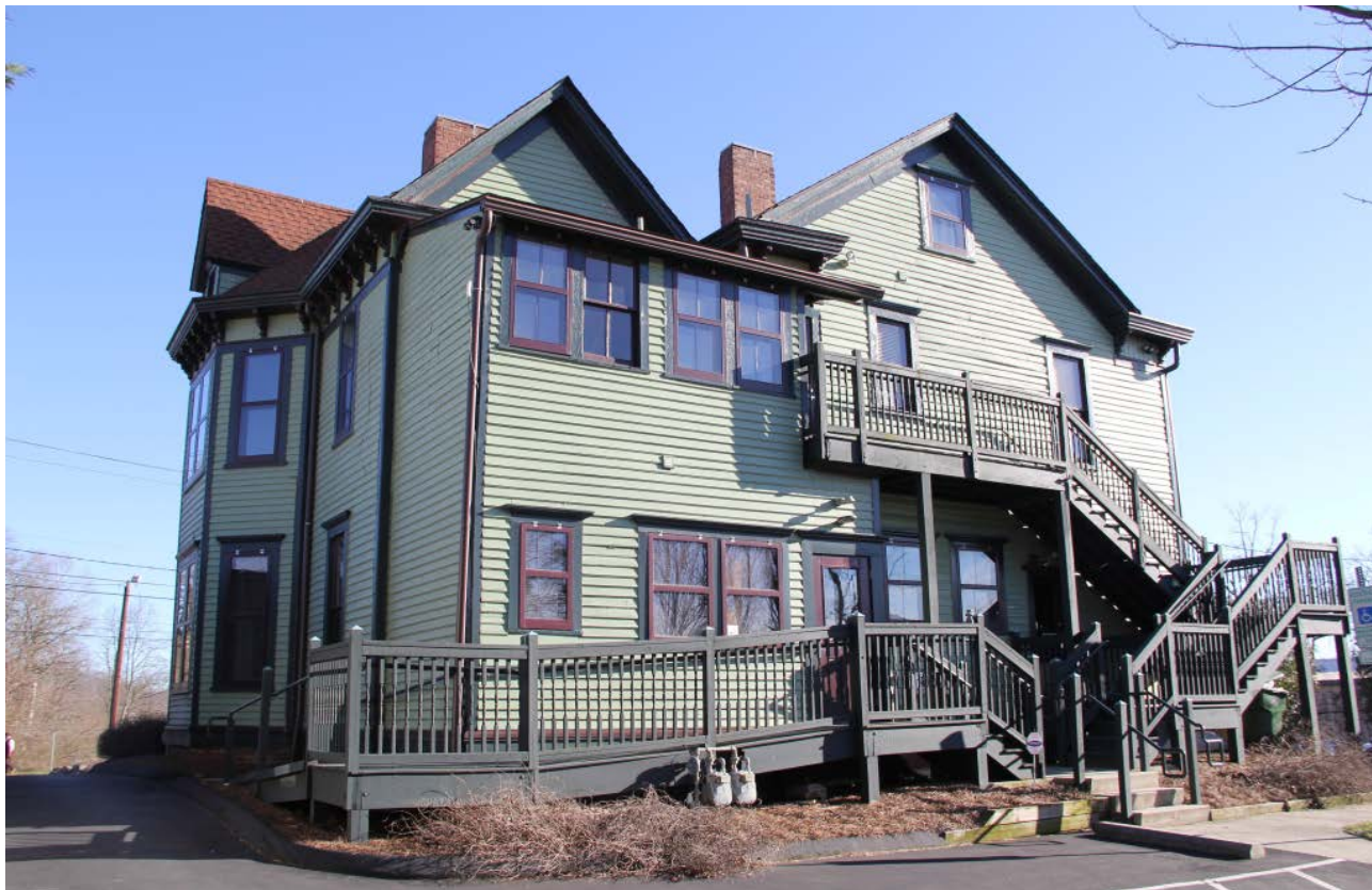
Whiteford G. Smith House, rear elevation, view to south
