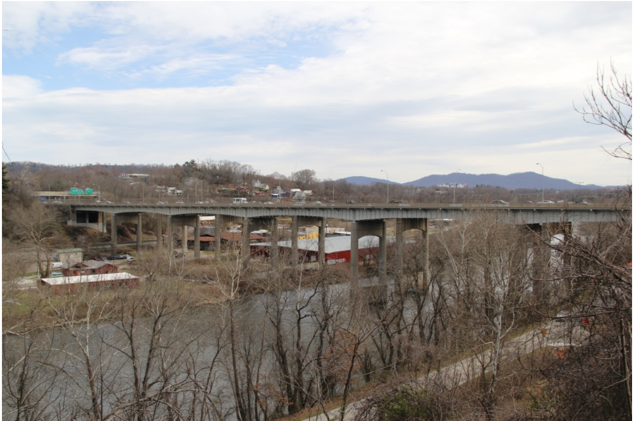
Great Smoky Mountain Park Bridge, view to southeast across Emma Road
