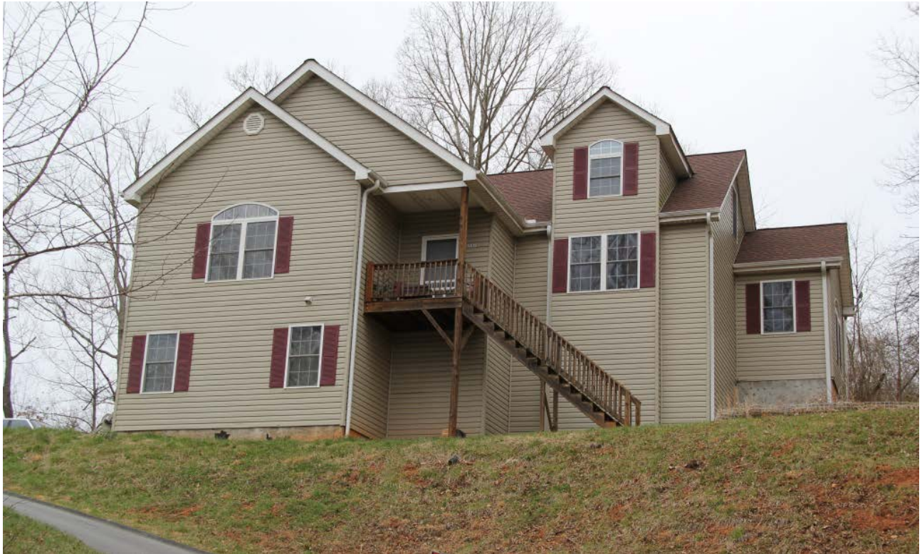
Payton House, built 2008, 341 Pearson Drive, view to northwest (excluded from boundary expansion)
