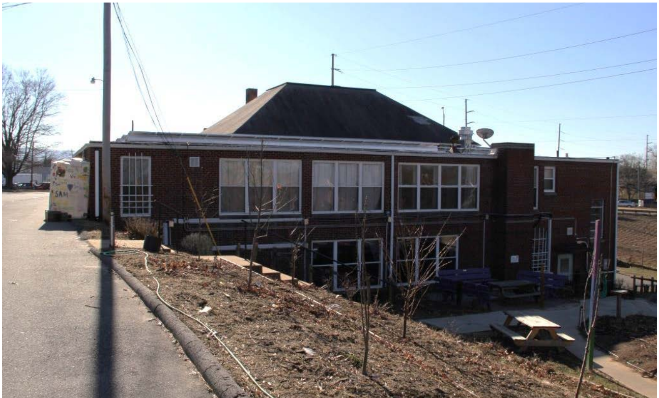
Haywood Street United Methodist Church, rear wing, view to southwest
