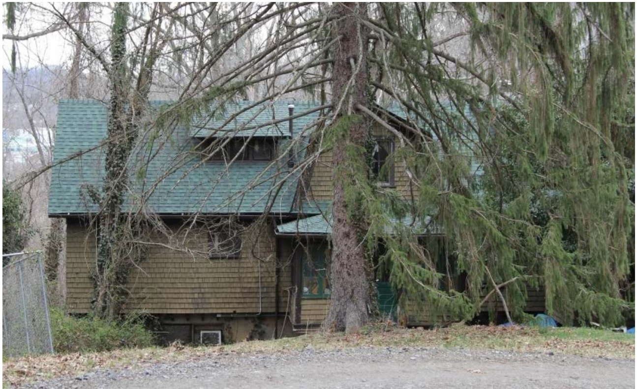
Hapke House, 72 Hibriten Drive , view to northwest
