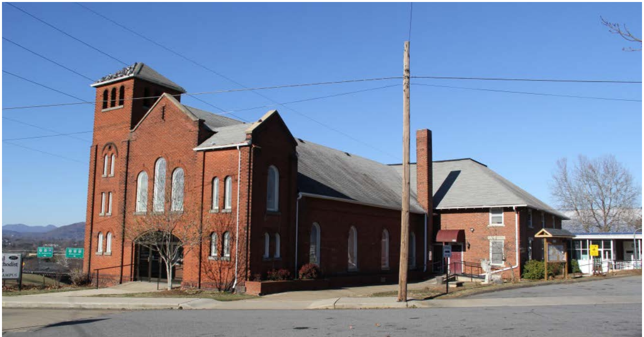
Haywood Street United Methodist Church, 297 Haywood Street, oblique view to northwest
