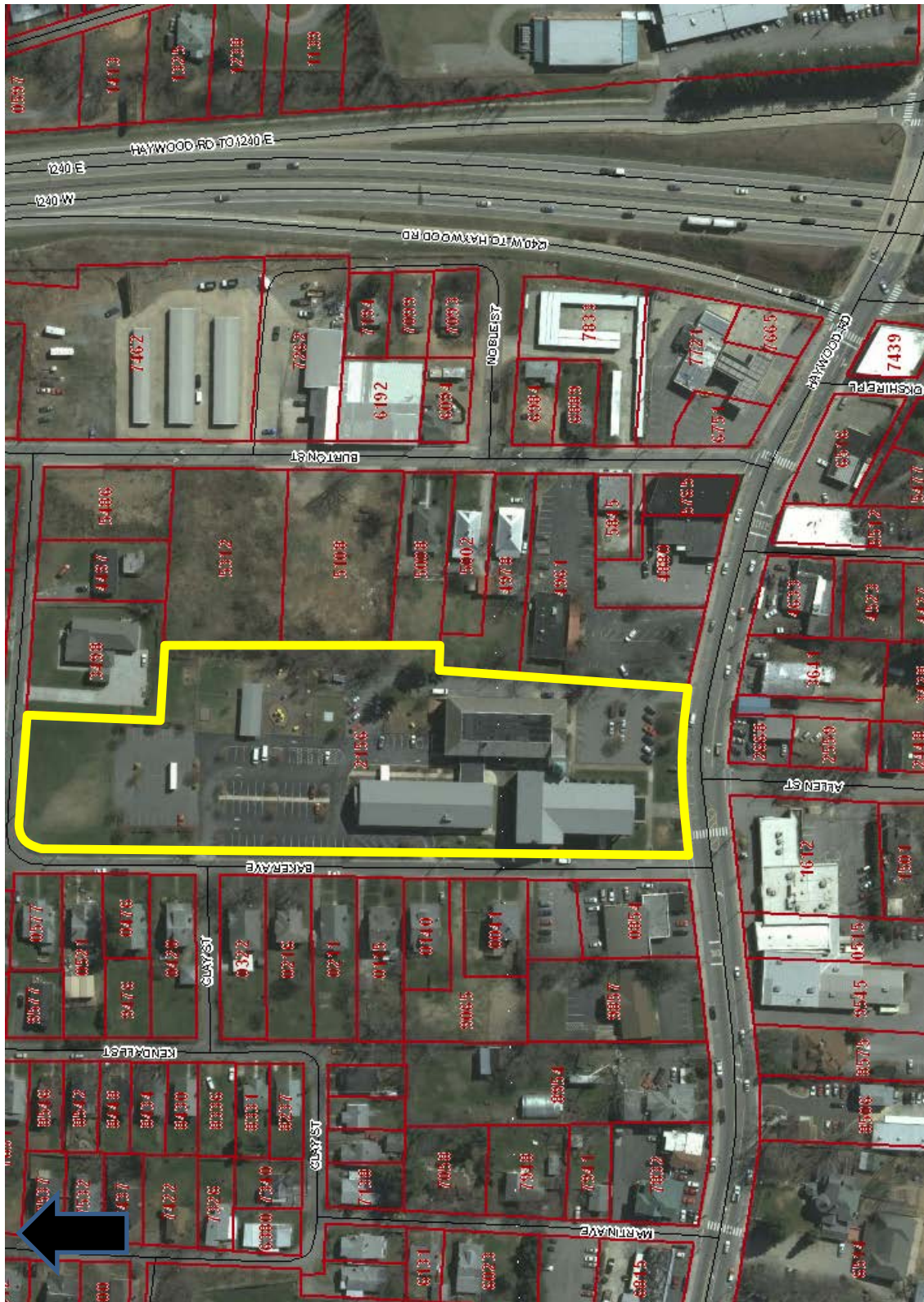
Calvary Baptist Church (BN4921), 531 Haywood Road [PIN 9638-45-2156-00000] (Map source: Buncombe County GIS)
