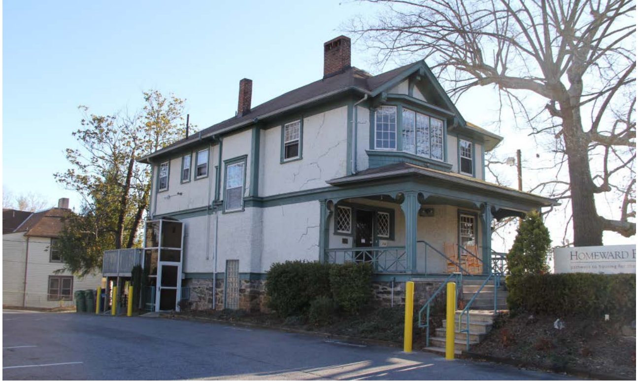
Mrs. Minnie Alexander Cottage, oblique view to southwest
