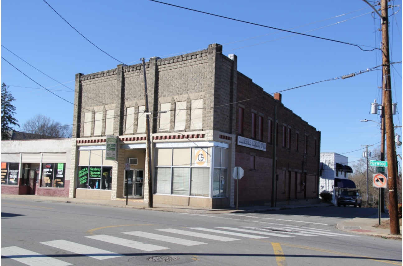
Baker Building (former Friendly Grocery Store), 503-505 Haywood Road, view to northwest
